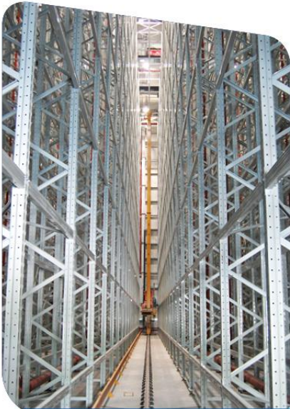
货架系统 Racking System
